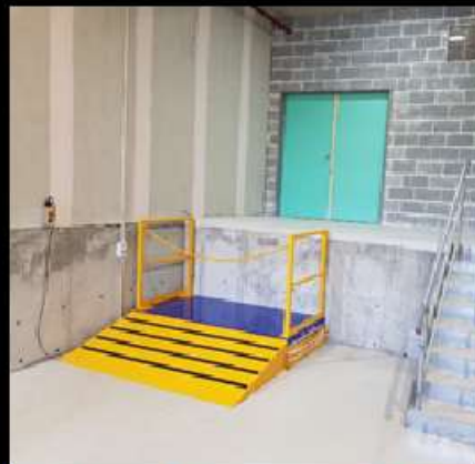
TQM Cahill Gardens Wollie Creek project - Wheelie Bin Lifter
